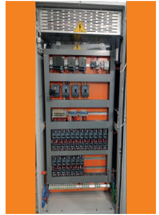
Motor Control Panel
